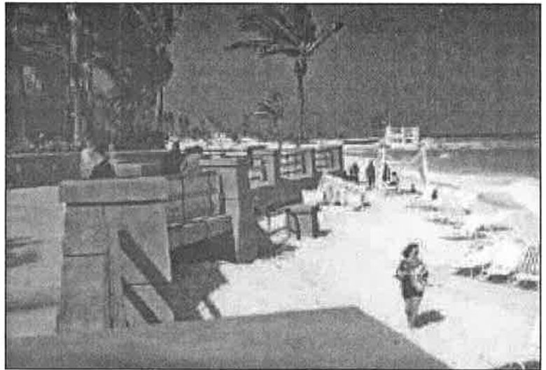
Figure 3. Landward relocation of Atlantis infrastructure away from the active beach, after Hurricane Floyd.
